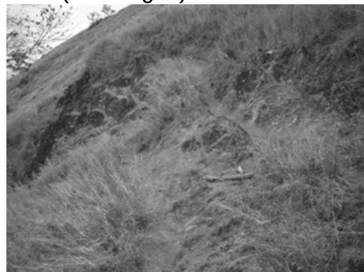
Picture 4: Erosion on a deforested mountain slope (Santa Lucia).
