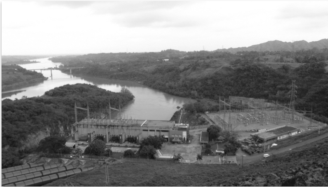
Figure 11: The S.N. Aboitiz power plant (photo by JR, 2011)
