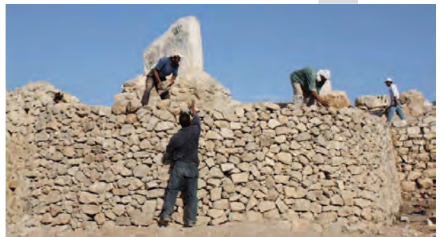
Figure 8.10 Rebuilding of the retaining wall.
