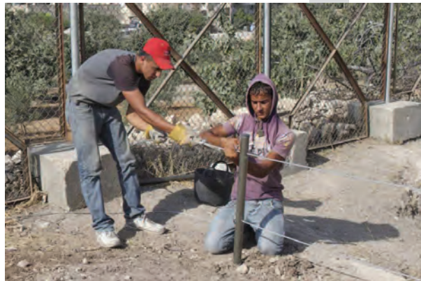
Figure 8.12 Maintenance of a fence.
