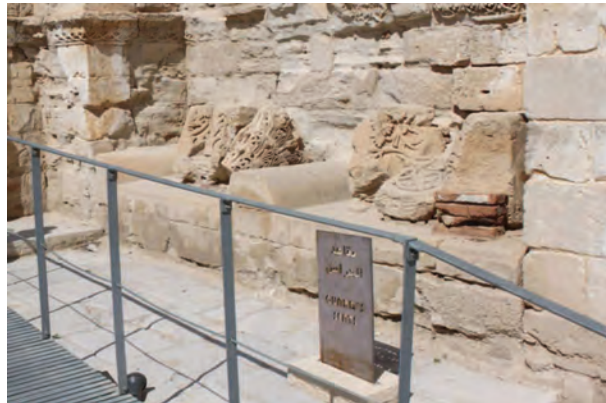
Figure 2.2 An example of protection at Hisham's palace, Jericho.
