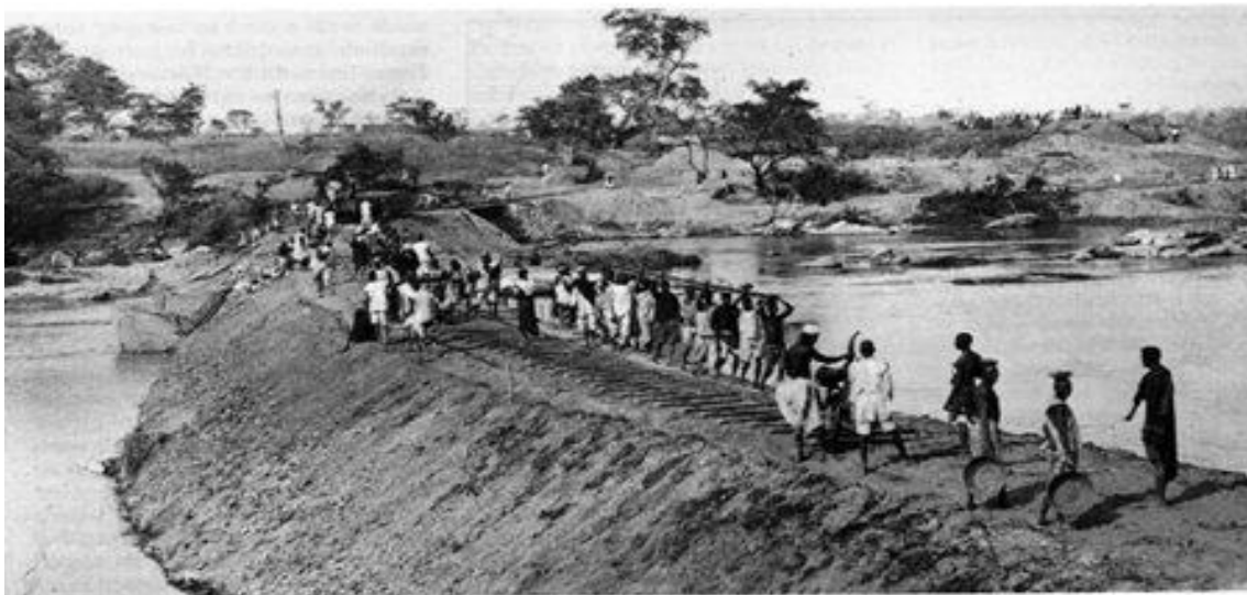
Figure 2.9 Construction work near Kaduna in 1910
