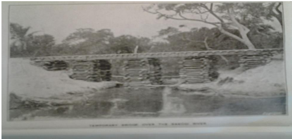
Figure 2.7 Temporary bridge over the Bakogi River
