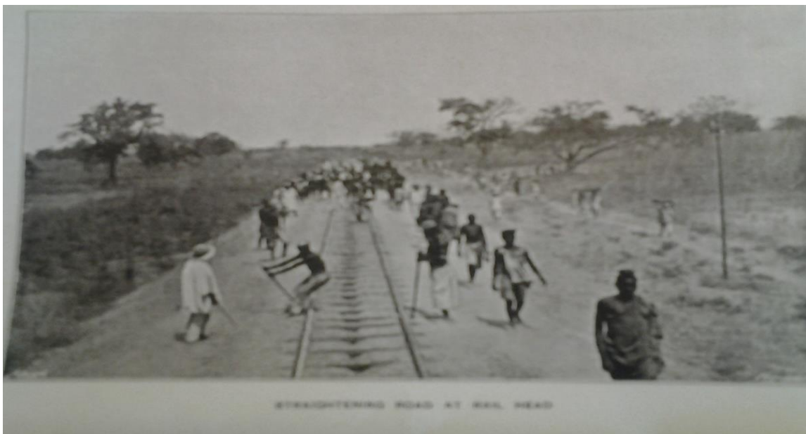
Figure 2.10 Construction work near Kano
