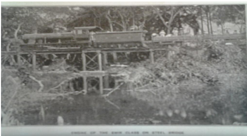
2.8 Testing of the Emir Class engine on a steel bridge
