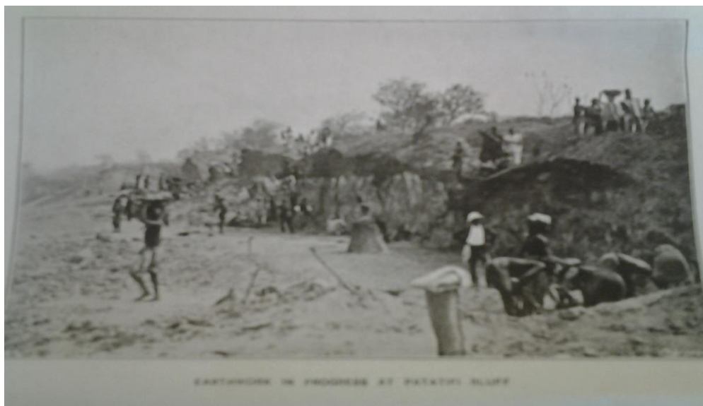
Figure 2.2 Earthworks in progress at Patatifi Bluff
