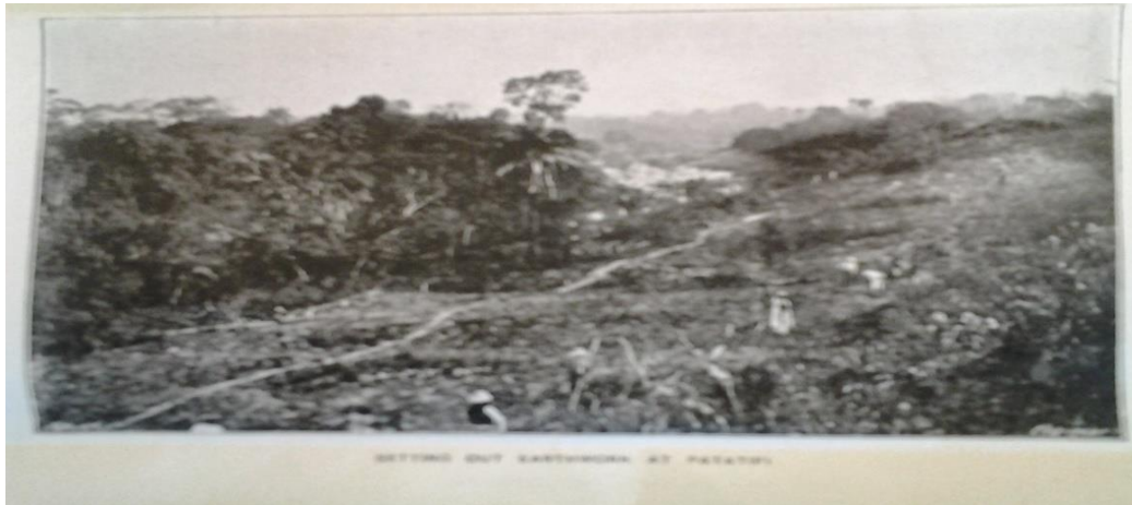
Figure 2.1 Setting out for earthworks at Patatifi
