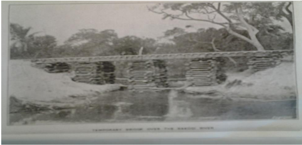
Figure 2.7 Temporary bridge over the Bakogi River
