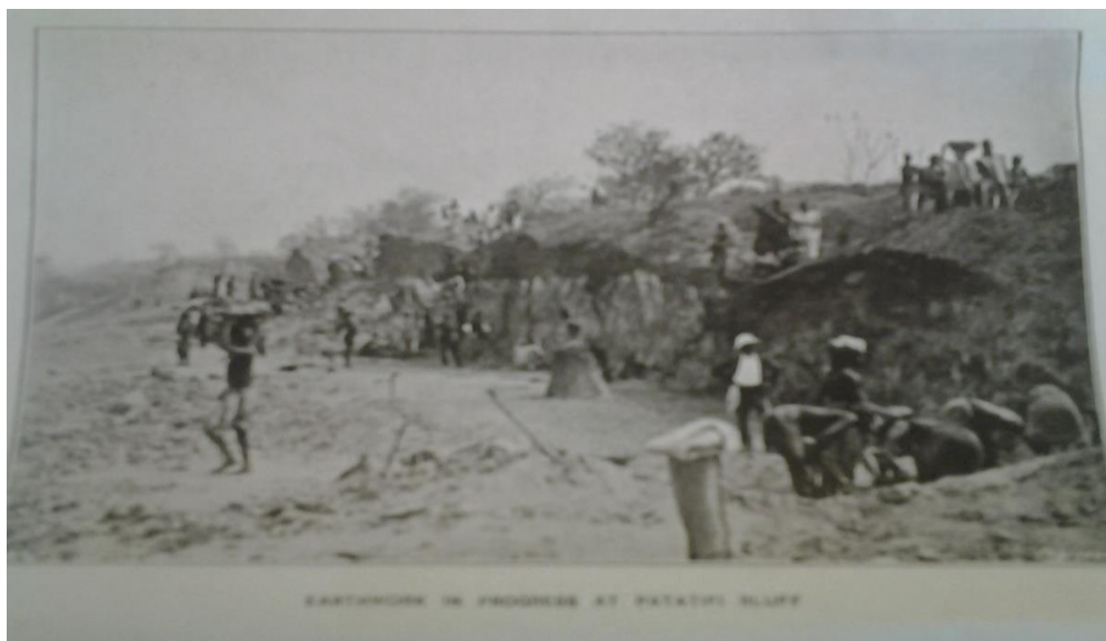
Figure 2.2 Earthworks in progress at Patatifi Bluff
