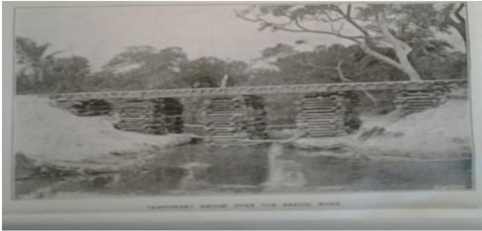
Figure 2.7 Temporary bridge over the Bakogi River
