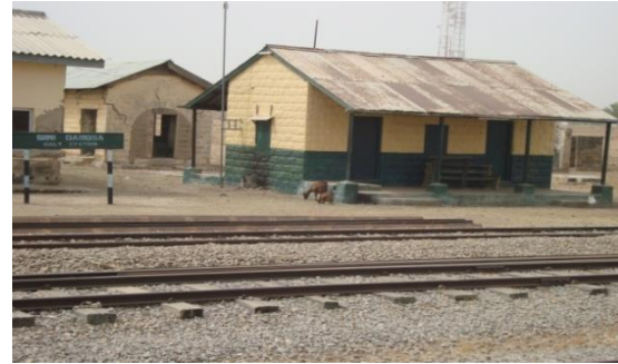
Gimi Dabosa Station
