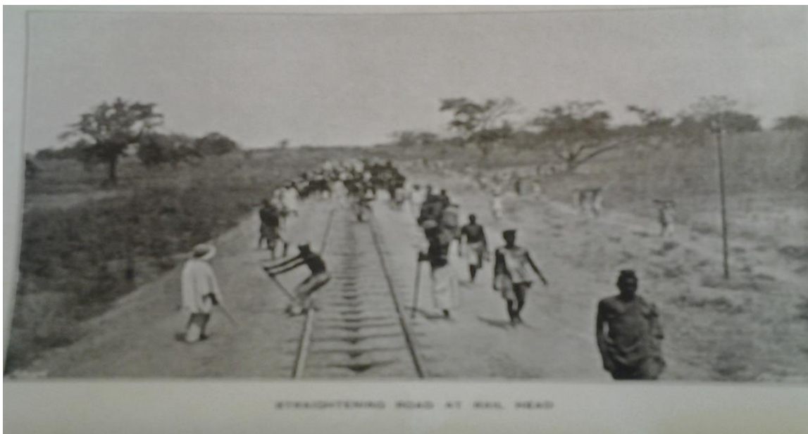
Figure 2.10 Construction work near Kano
