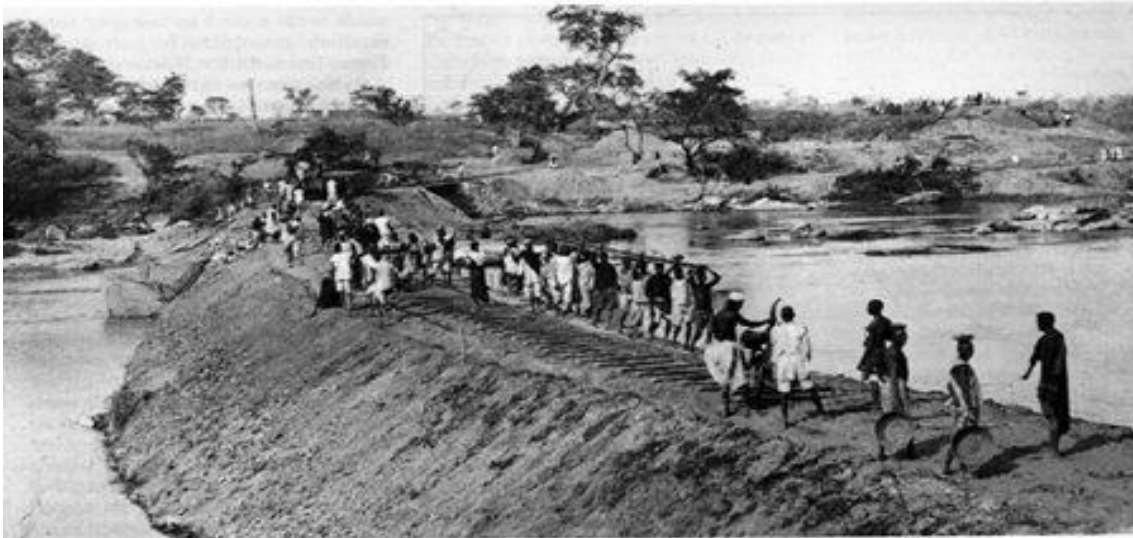
Construction of the Kano-Lagos railway in process near Kaduna in 1910.
