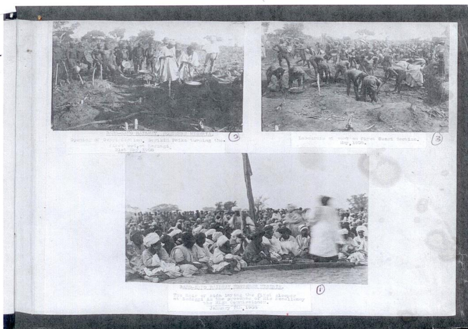
Figure 2.4 Railway construction in Nupe Province
