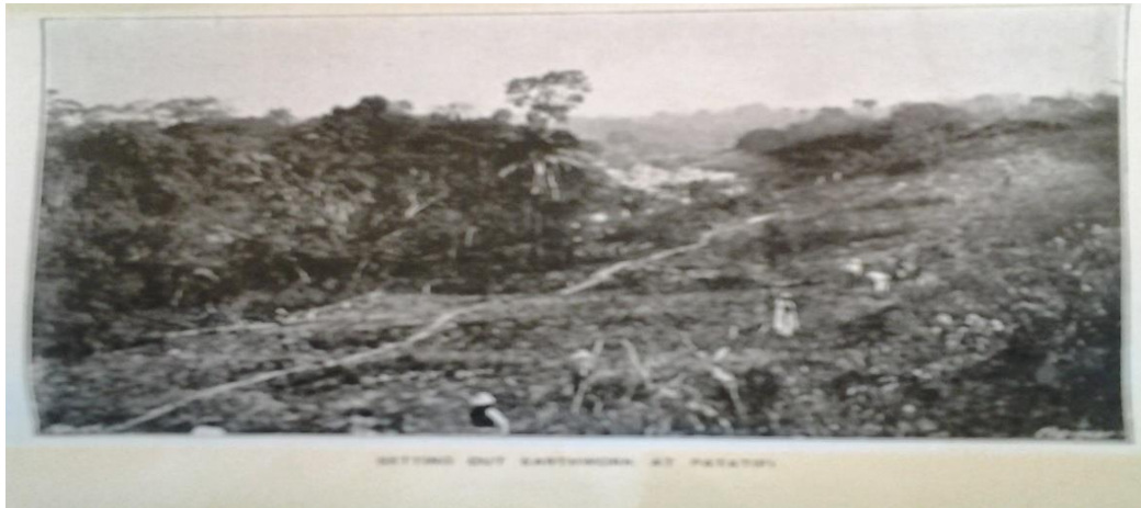
Figure 2.1 Setting out for earthworks at Patatifi
