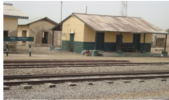
Gimi Dabosa Station
