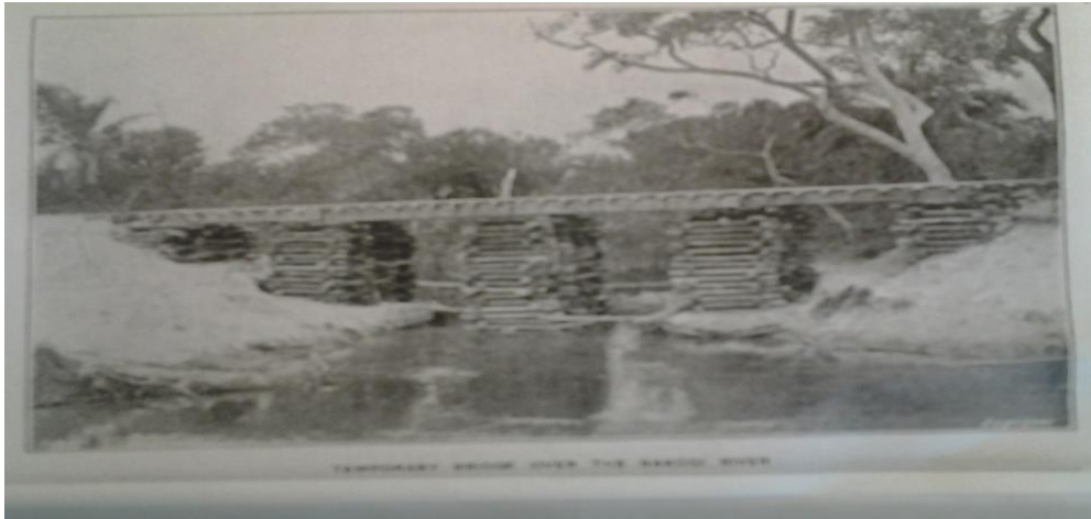
Figure 2.7 Temporary bridge over the Bakogi River
