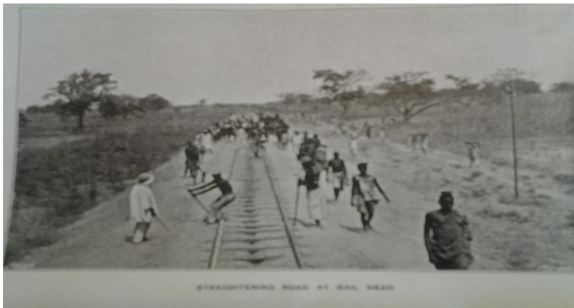
Figure 2.10 Construction work near Kano
