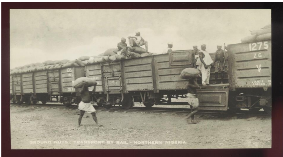
Figure 6.2 Open groundnut wagons
