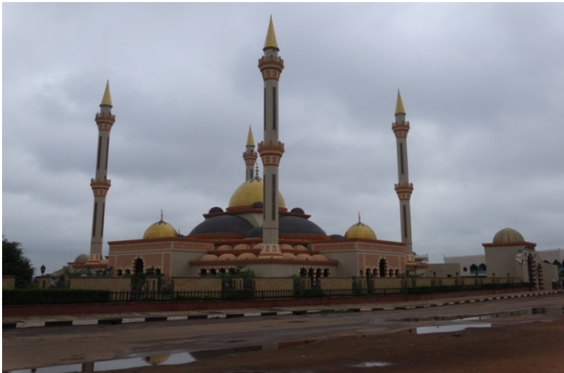
Fig. 29. Ilorin Central Mosque refurbished in 2012. Picture taken by the researcher, 2014.
