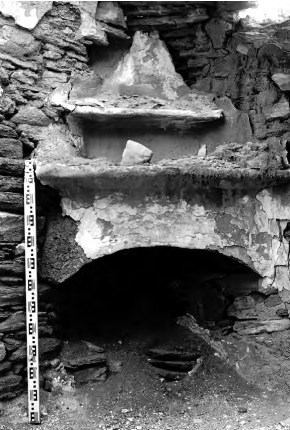
Fig. 6.101 Low corner-hearth in a house at Ismaili
