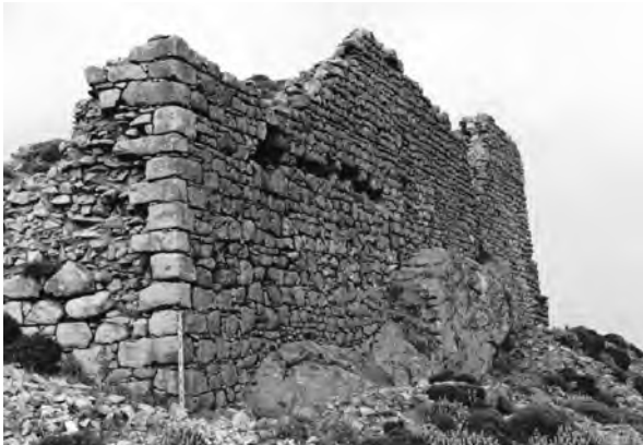
Fig. 6.25 View of Hall A from the Northeast with a long gap on the stone masonry suggesting the position of the wooden balcony-like projection
