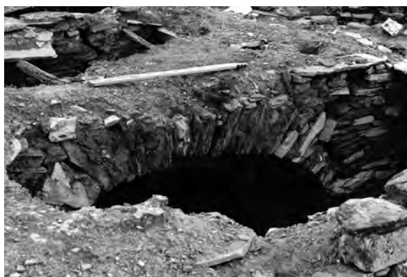
Fig. 6.99 A collapsed roof supported by an internal stone-built arch in a house at Ismaili
