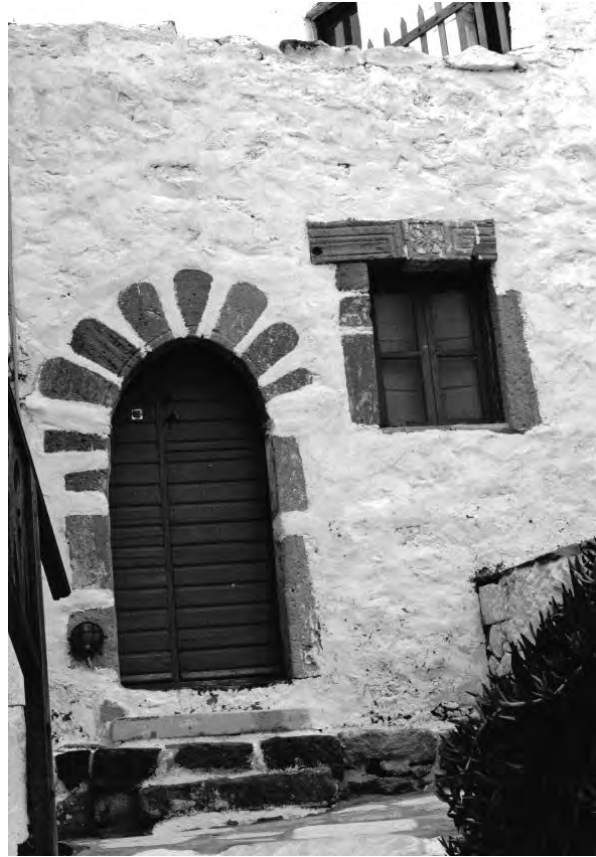
Fig. 6.62 View of a house from Kastro with decorative stone-frames and lintels
