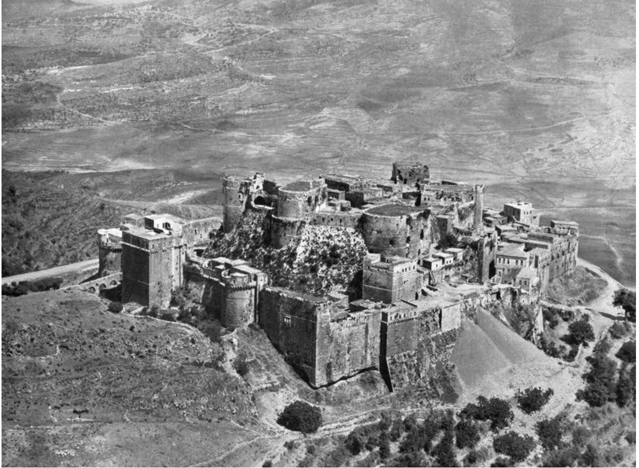
Fig. 4.7 Overview of the castle of Crac des Chevaliers. Müller-Wiener 1966.
