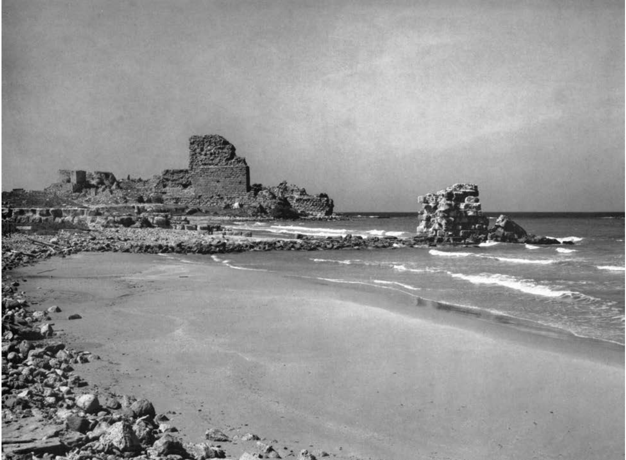
Fig. 4.16 'Atlit, view from the (nowadays inaccessible) shore side. From Müller-Wiener 1966.
