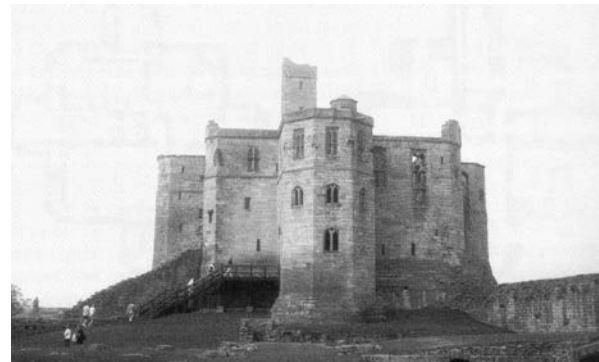
Fig. 6.7 Warkworth castle in Northumberland, frontal view. From Johnson 2002.
