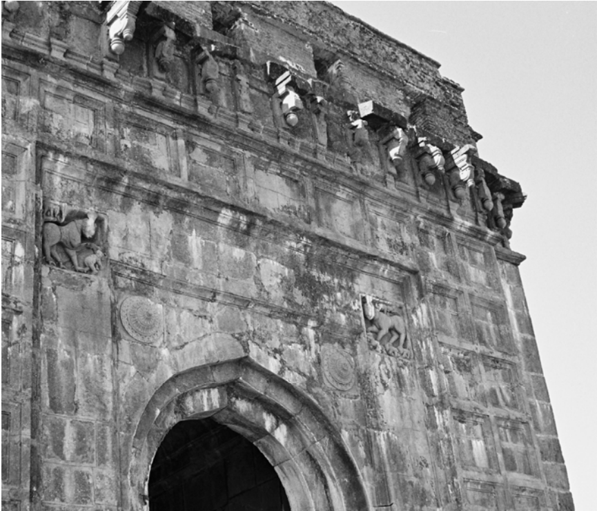
East face of the gate to the ceremonial core of the Raigarh fortress.
