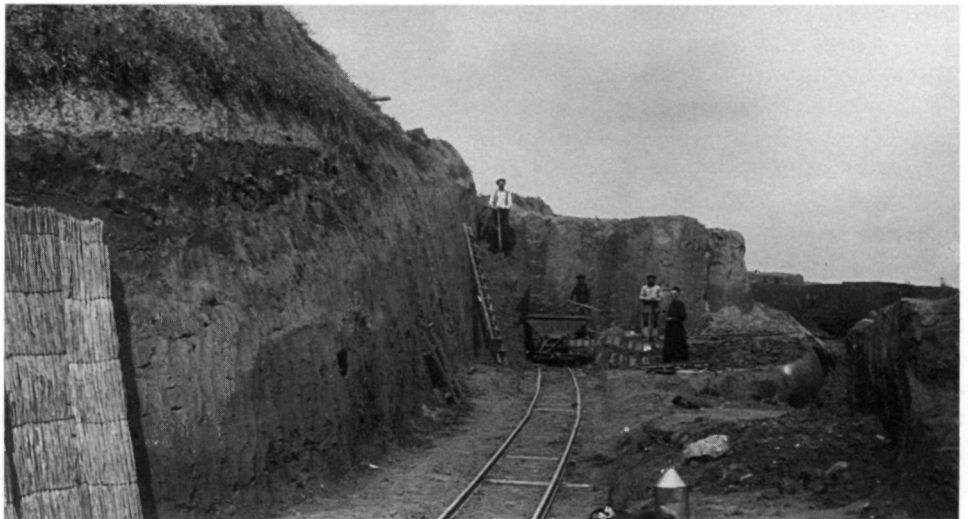
Fig. 6. A, B and C. The Belvédère pit: photographs taken in the 1930s (Municipal Archive of the city of Maastricht).
