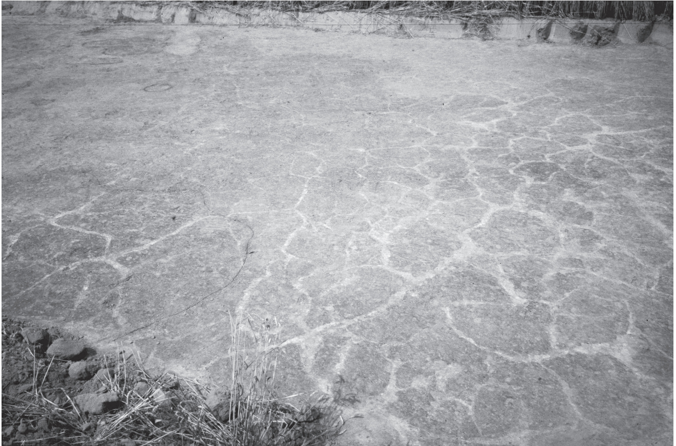
Fig. 3.5 Field photo of desiccation cracks.
