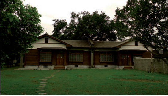
Fig. 4.4.2 Building F, a semi-detached residence, is the only renovated one among the Jiangjunfu residences. Photo was taken in April 2011 by the author.
