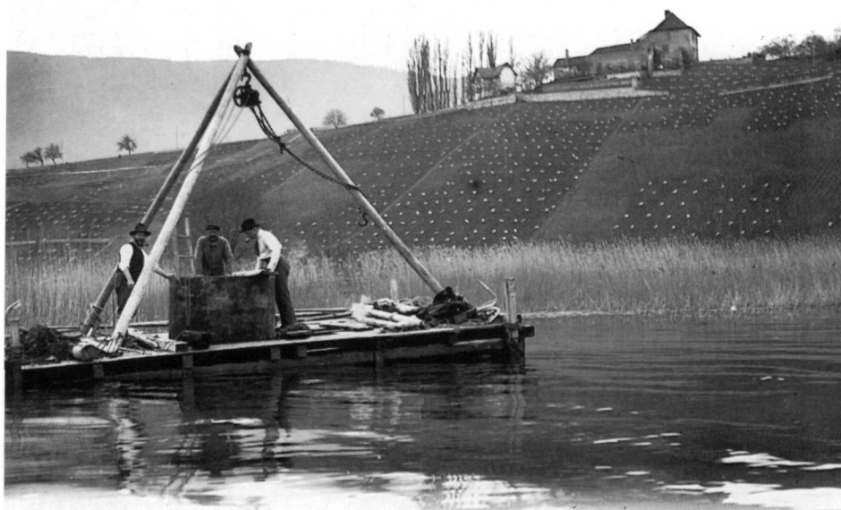
Figure 7. The logical extension of the European tradition of archaeological field-research beyond the limits set by the waterline. Paul Vouga uses a three meter deep caisson for test excavations at the late Bronze Age settlement of Cortaillod in the spring of 1925 (courtesy Archives du Musée Cantonal d'Archéologie, Neuchâtel).
