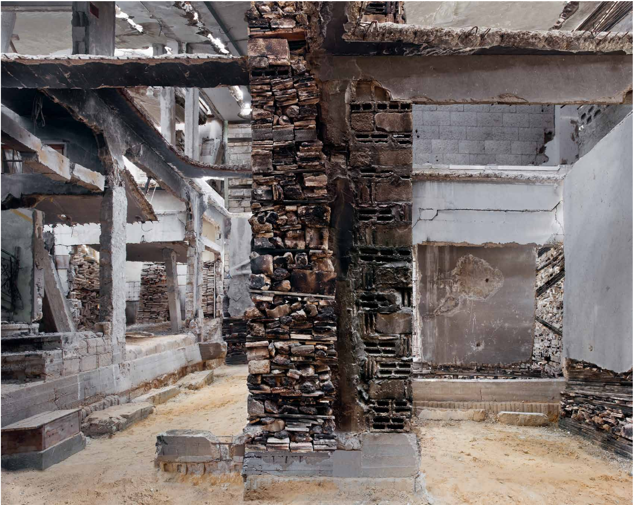
Destroyed House Gaza 14
