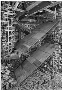
p. 47 Destroyed House Leiden 3 , Leiden (NL), 2016, 221.5×155 cm, inkjet print on dibond/framed
