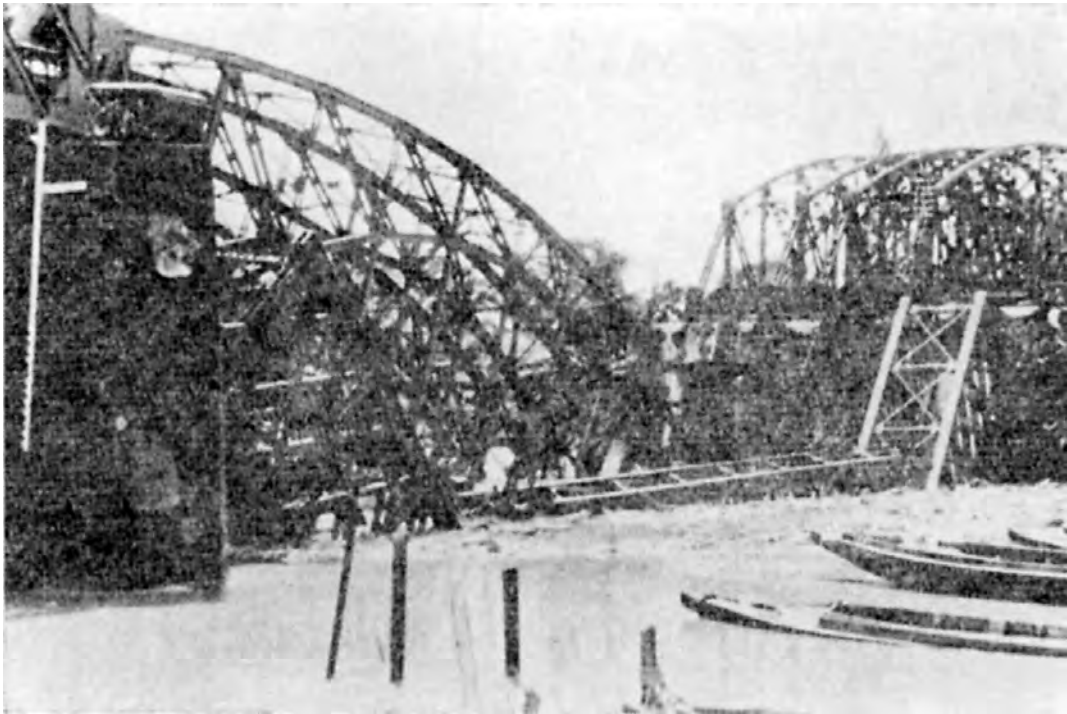
The Destroyed Bridge at Kragilan
