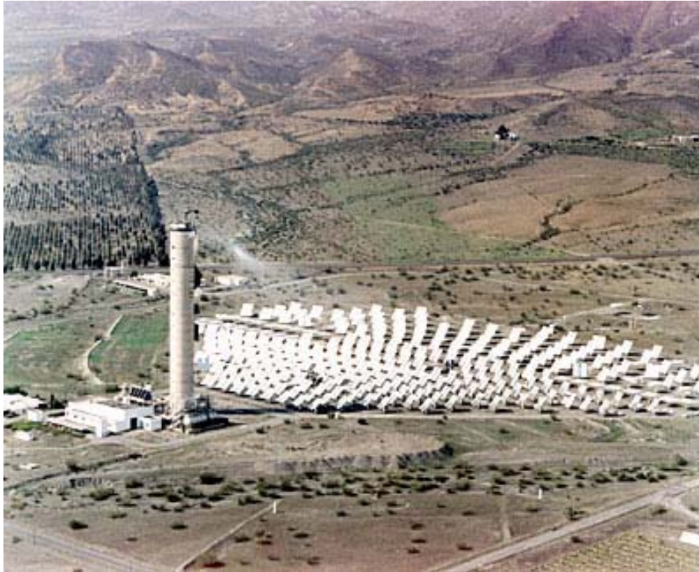
Figure 5. Solar Tower plant in Almeria, Spain.
