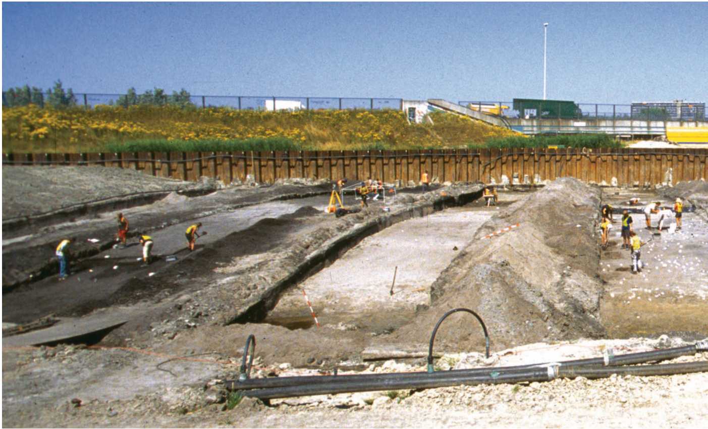
Figure 1.7 General view of the site from the south, half way through the excavation.
