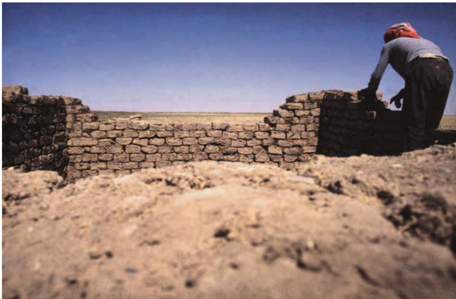
Figure 5 A modern builder concentrates on the corners of the walls.
