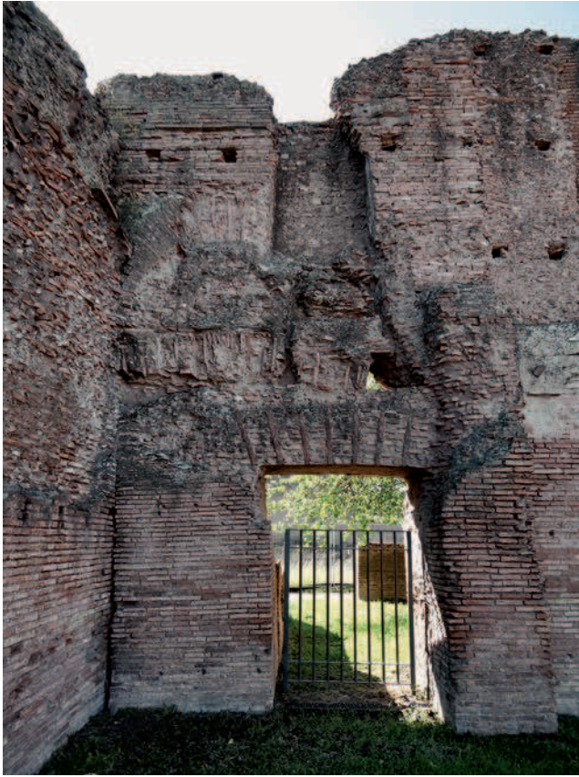
Figure 5 Entrance to room 533S, seen from the west: The existing entrance is a later reduction of a wider opening from the original building phase. The changes can be deduced e.g. from the remains of the relieving arches. Photo L.C. Götz.
