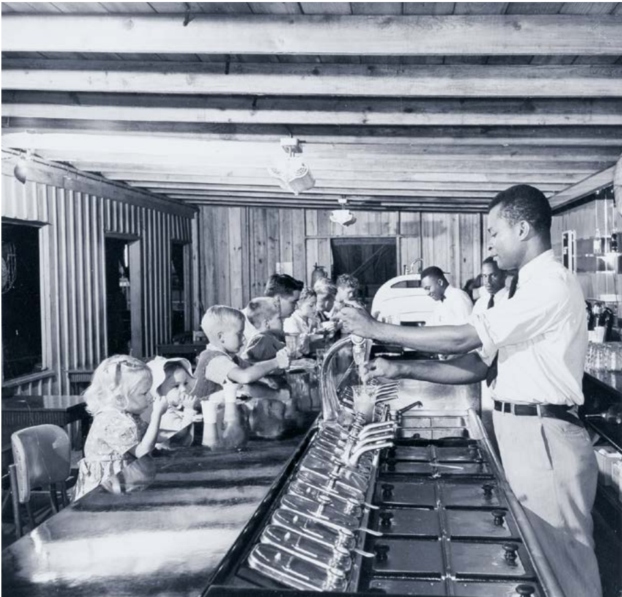
A separate residential neighborhood was built for the Dutch, European, and American employees of the oil refinery in Aruba. Its social center, called the Esso Club, boasted all sorts of facilities, including an ice cream parlor. The photo shows Black employees serving the children of Esso’s white employees.
