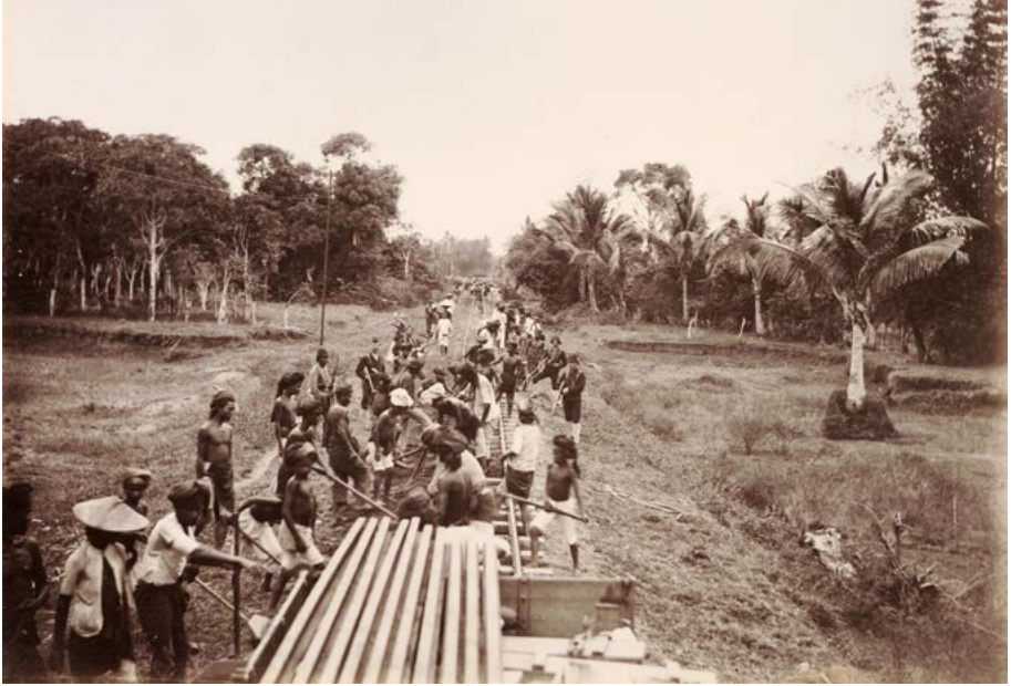
This photo, which was taken in 1905, shows forced laborers repairing the railway used by the Aceh tram near Meureudoe. Soldiers armed with rifles can be seen supervising the workers.
