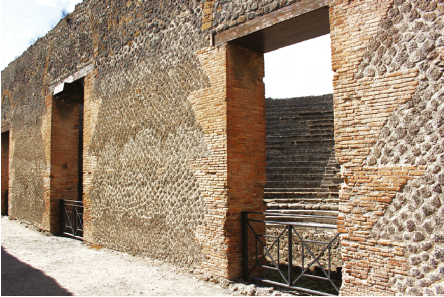
FIGURE 7.6 Pompeii, Odeon: early colonial opus incertum with grey lava and brick PHOTO: MIKO FLOHR
