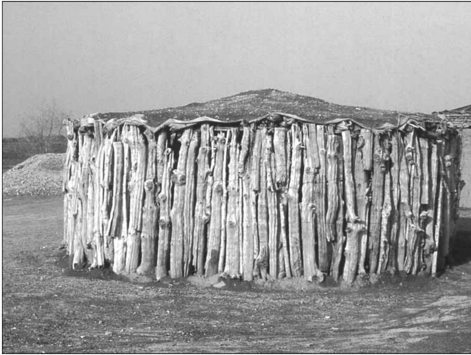
Figure 5-7: A Hadendowa dwelling made of Euphorbia stems in northeast Sudan, near the Egyptian border.
