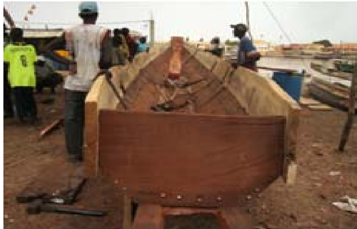
Construction of a Pirogue
