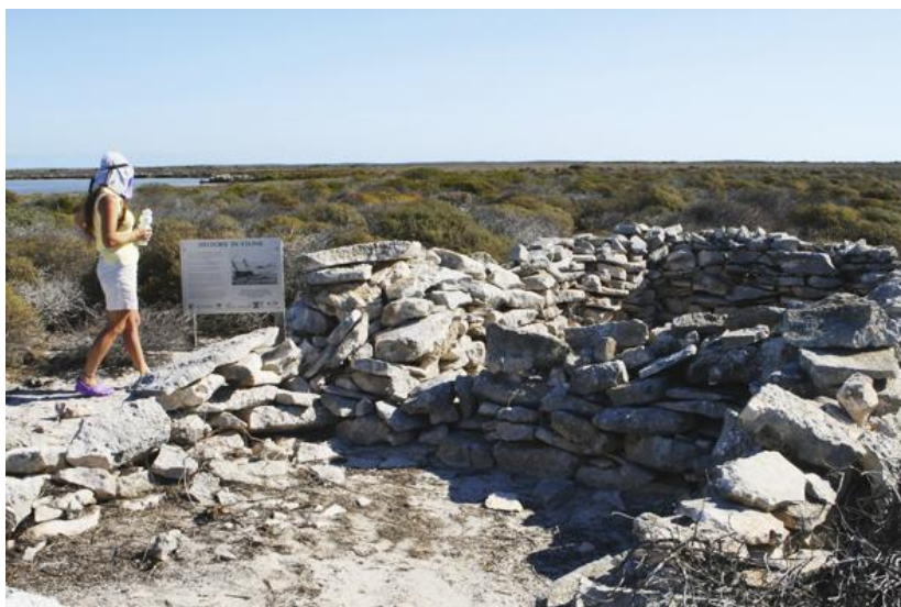
Figure 20: Coastal structure, Slaughter Point site
